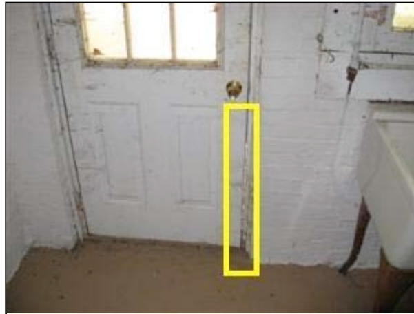
2.1 Picture 1 Basement entry
