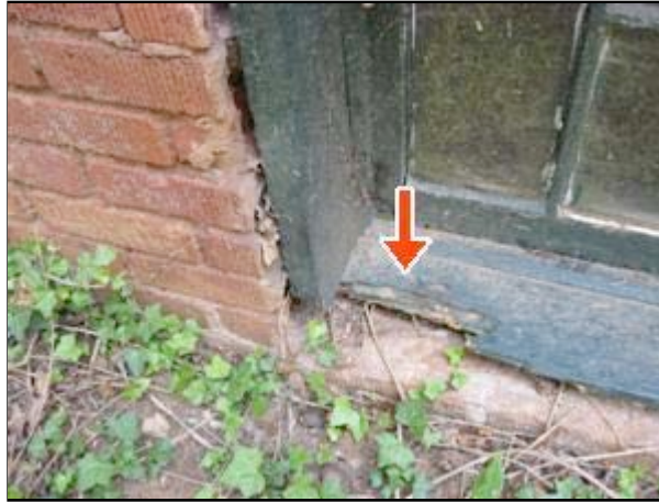
2.2 Picture 1 Basement window (s)
