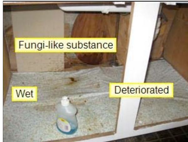
3.4 Picture 1 under kitchen sink
