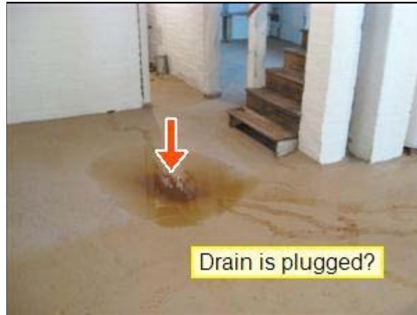
5.0 Picture 4 basement floor drain
