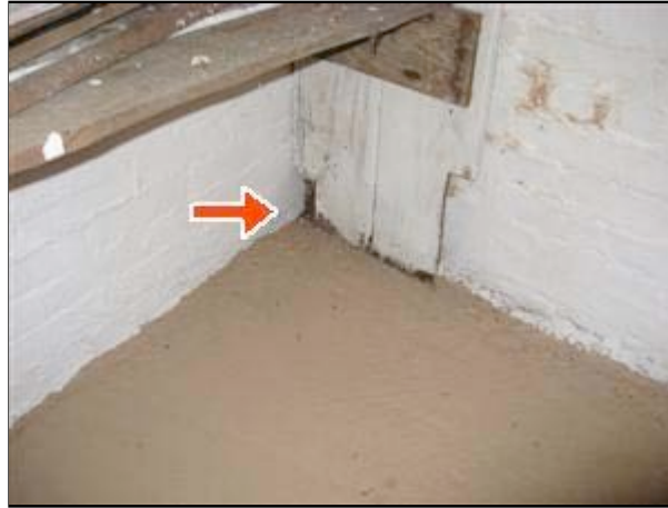
4.0 Picture 2 basement wall
