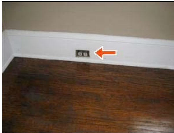
6.3 Picture 1 various rooms
