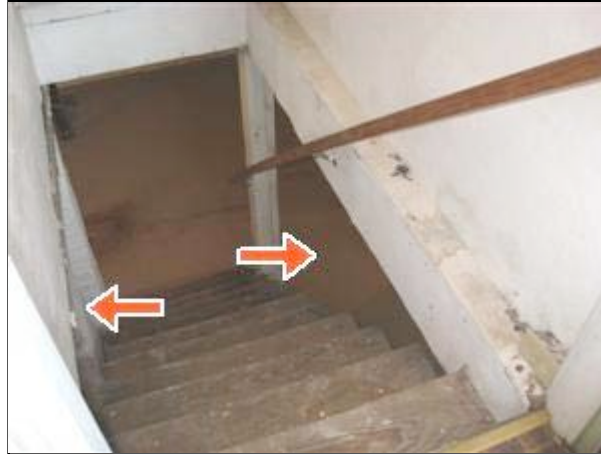
3.3 Picture 1 basement stairs
