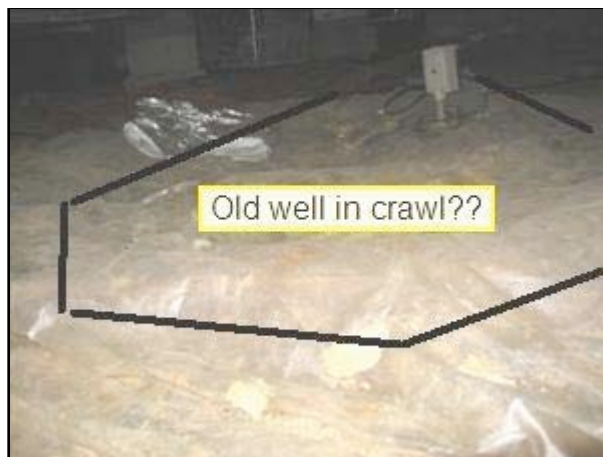
2.6 Picture 2 in crawlspace under new addition
