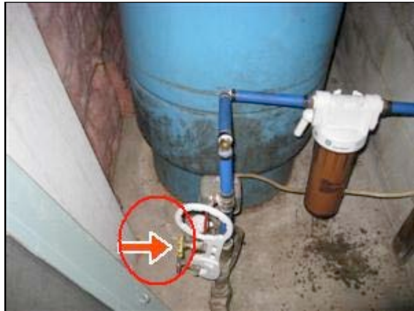
4.3 Picture 1 In basement
