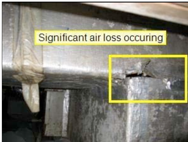
6.3 Picture 4 crawlspace new addition
