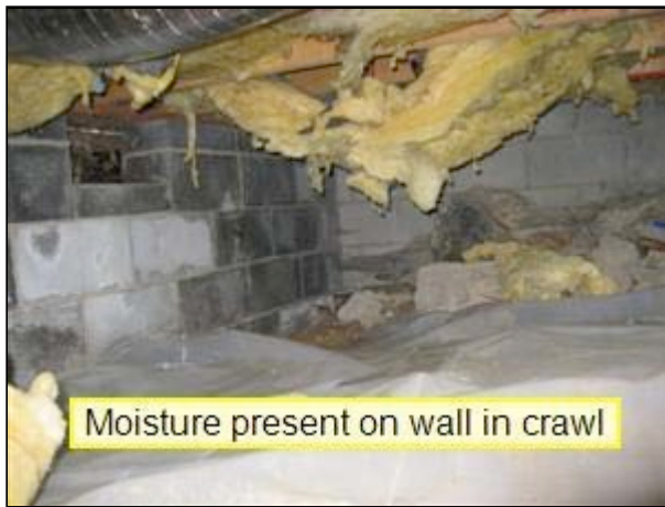
1.0 Picture 5 crawlspace under kitchen
